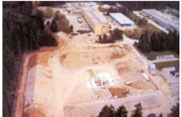
Fig. 1. Building-up of P 59 with safety walls.
